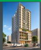
Business Tower Kalshi · 2030
